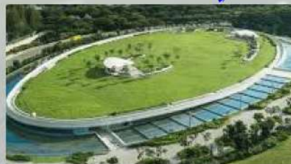
Marina East Desalination Plant
